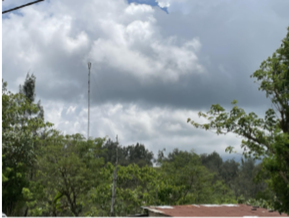
Mobile tower in Malilait village (Bobonaro)
